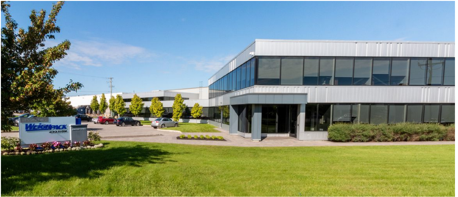
Paxiom Group's WeighPack manufacturing facility in Montreal is one of the company's biggest production sites worldwide.
